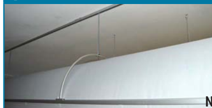
External Arch profile [track] hanger [N]
