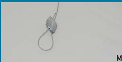
Gripple hangers - lower part [M]
